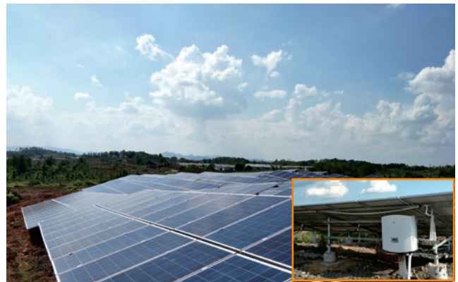
Jiangxi Ganzhou PV Plant 3.5MW
