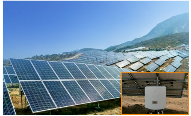
Liaoning Yingkou Jiuzhai PV plant 20MW
