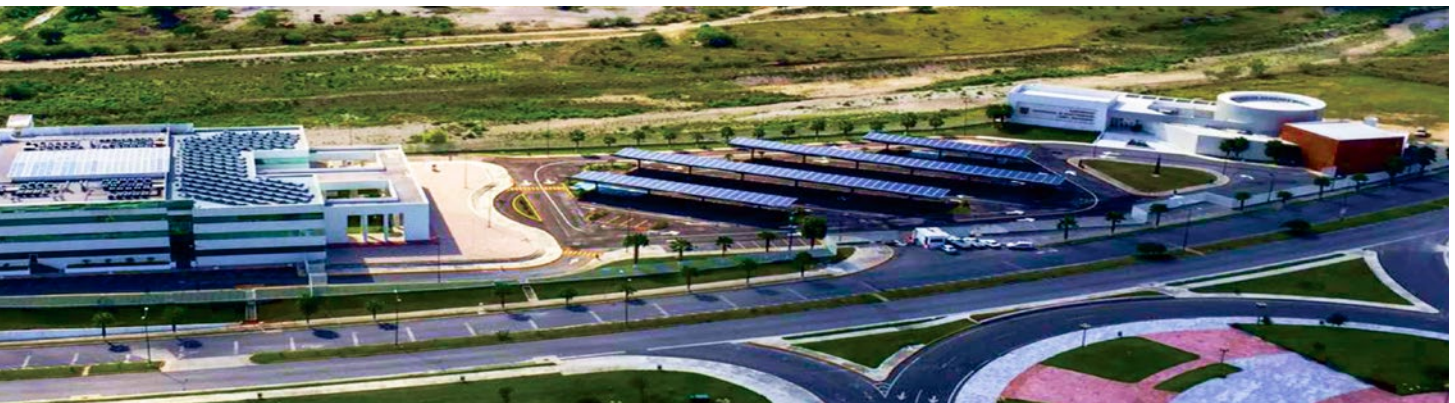
Mexico-Tamaulipas Carport, Mexico 5MW
