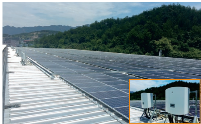
Hainan JiuLongGlass 1.7MW
