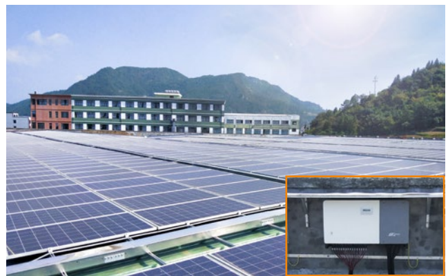
Tyco Electric, Panan Jinhua Zhejiang 1.5MW
