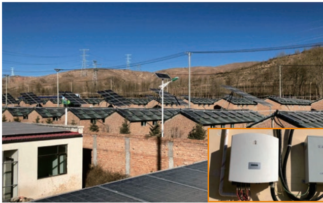
Qinghai HuzhuBanyan poverty alleviation PV Plant 2MW
