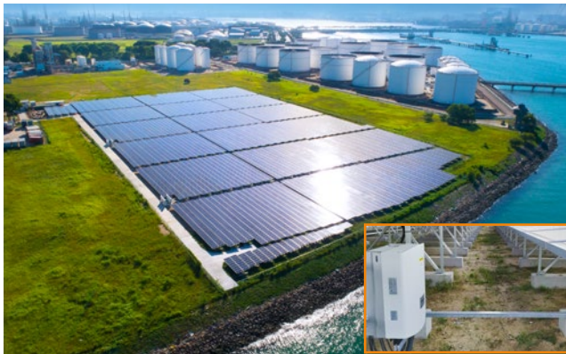
JTC Solar Farm, Singapore 5MW
