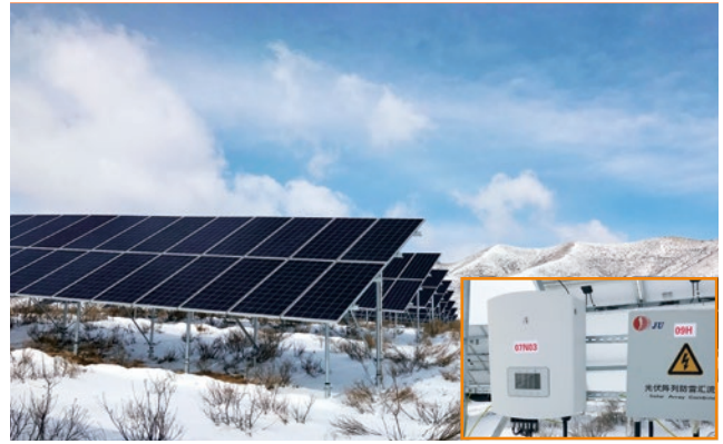
Shanxi Guangling PV plant 1.47MW
