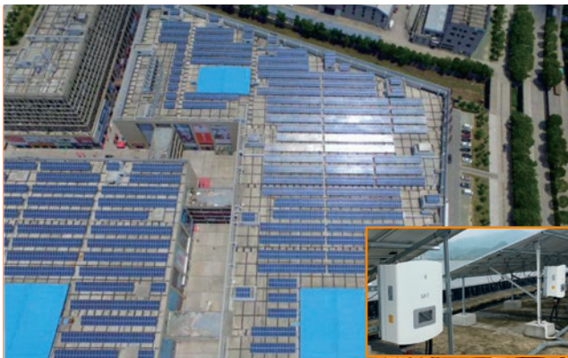
Ninghai AB hall, modern home plaza 1.53MW
