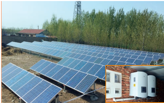
Shandong Leling poverty alleviation PV Plant 50kW
