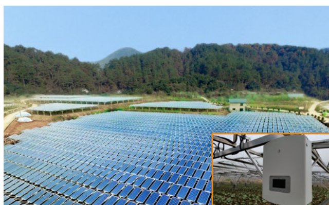
Zhejiang Dajie Agricultural-photovoltaic hybrid PV plant 3MW
