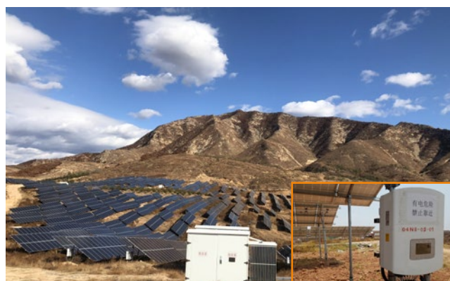
Liaoning Gaizhou Jiuzhai PV plant 20MW
