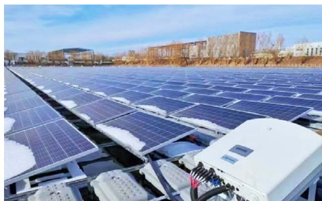
Beijing Shunzhen Green Harbor's Plant 5.5MW
