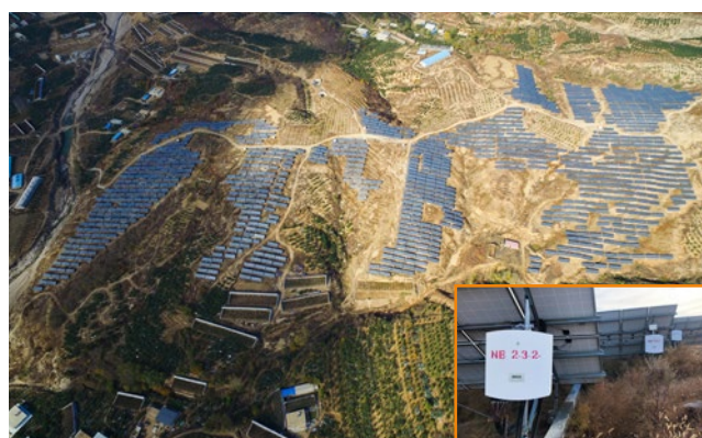
Liaoning Jiuzhai Gaizhou PV plant 20MW
