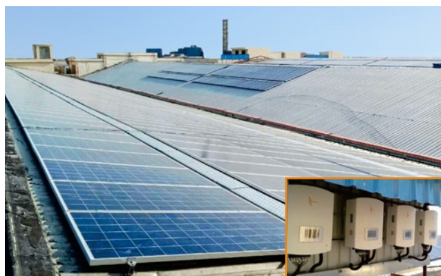
RSWM, India 3.6MW
