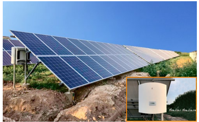
Hebei Qinghuangdao poverty alleviation PV Plant 5MW
