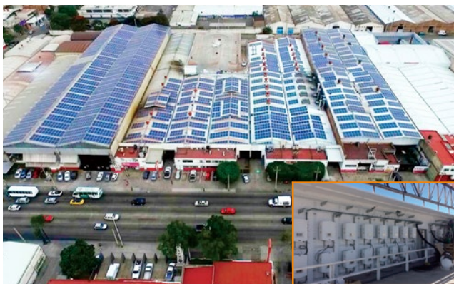
DEPSA, Mexico 3.4MW
