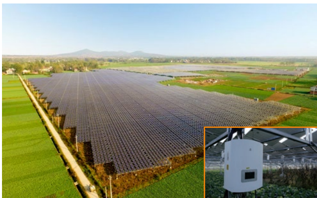
Hubei Guanyin Agricultural-photovoltaic hybrid PV plant 20MW
