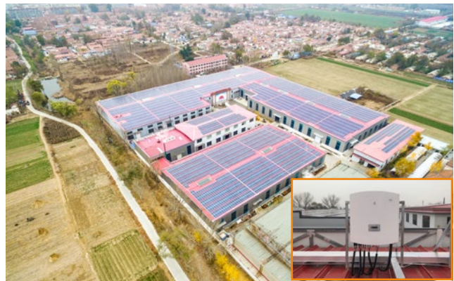
Shandong YUELONG 3.5MW
