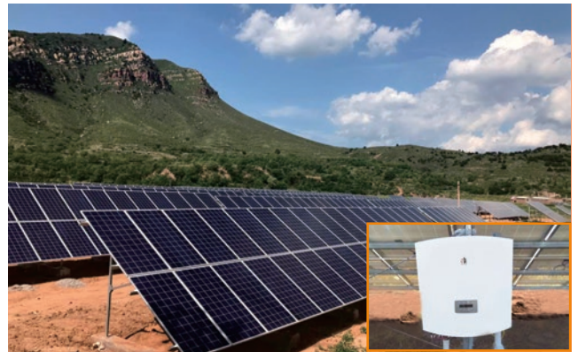
Shanxi Xiyang poverty alleviation PV Plant 7.2MW
