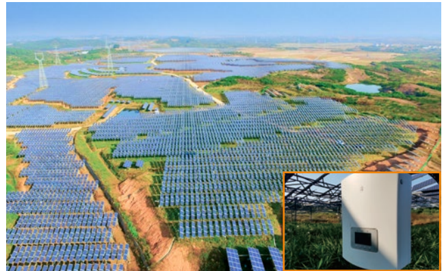
Zhejiang Hangbu Agricultural-photovoltaic hybrid PV plant 30MW
