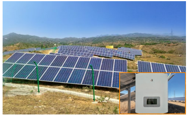
Hebei Qinghuangdao poverty alleviation PV Plant 9.7MW
