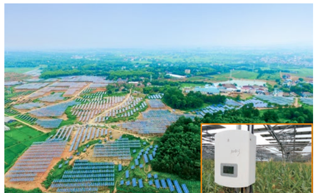
Quzhou Qinghu Agricultural-photovoltaic hybrid PV plant 20MW
