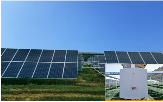
Hebei Zhangjiakou poverty alleviation PV Plant 5.1MW
