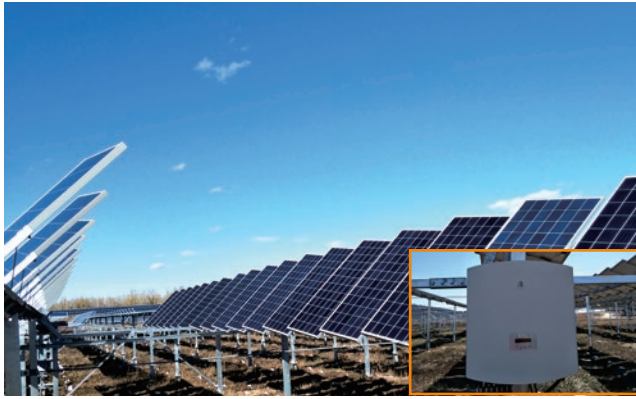
Hebei Zhangbei Agricultural-photovoltaic hybrid PV plant 50MW
