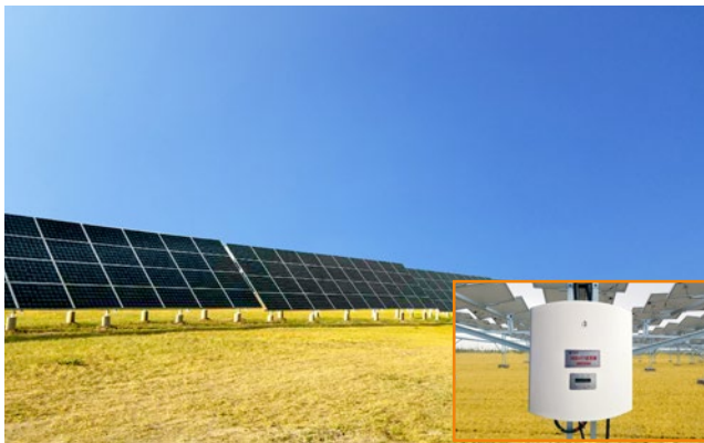
Huaneng Yimin surface mine PV plant 20MW
