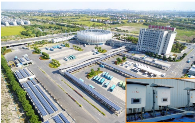
Zhejiang PINGHU Bus Station 472kW
